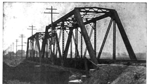
Typical Through Truss Bridge, Valley Route
