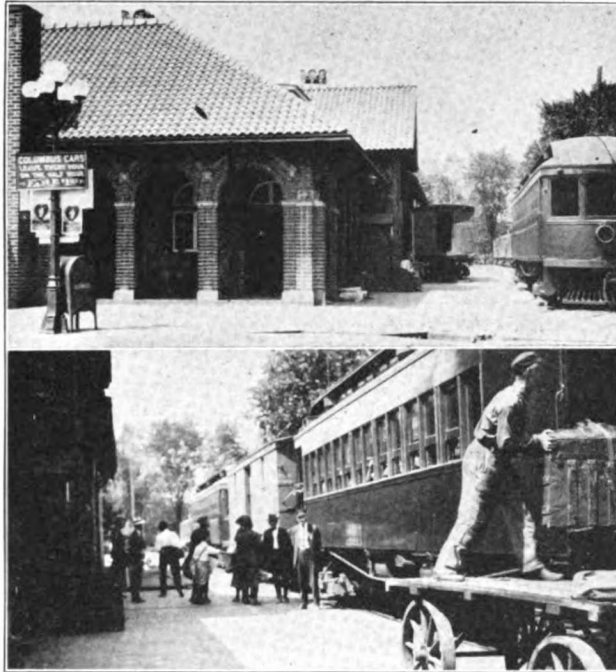
Upper View—Passenger and Freight Terminal, Chillicothe, Ohio. Lower View—Mixed Freight and Passenger Train Showing Method of Handling Rush Freight Traffic on Regular Passenger Run
