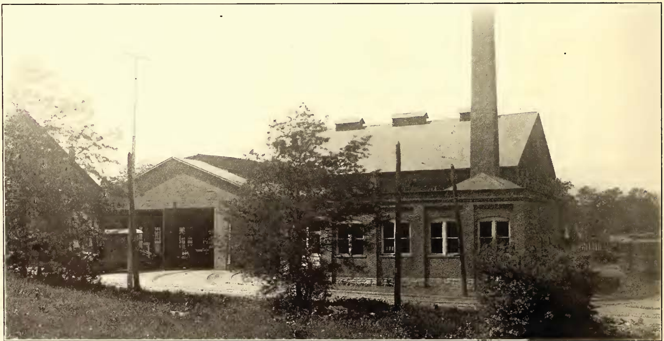
FIG. 1.—EXTERIOR OF REPAIR SHOPS, COLUMBUS RAILWAY & LIGHT COMPANY
