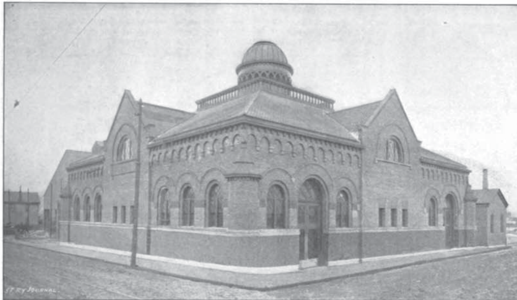
POWER HOUSE WITH CENTRAL STACK—COLUMBUS CENTRAL RAILWAY, COLUMBUS, O.
