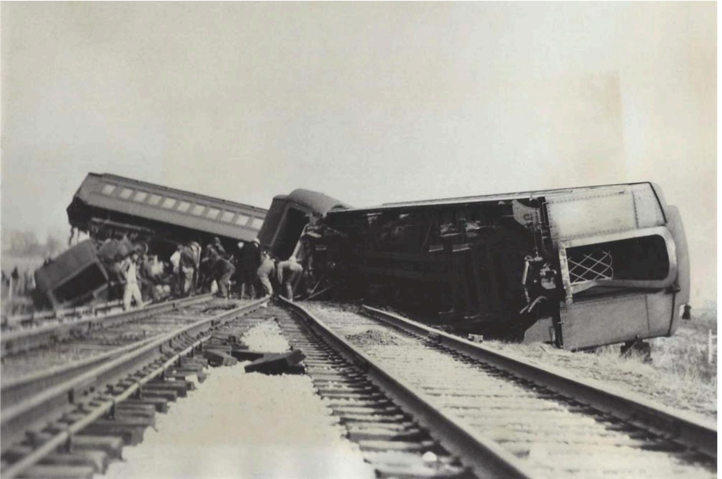
A press photo of the accident from the rear showing four derailed passenger cars and on the left between the two cars, the cylinders of one of the two steam locomotives.
