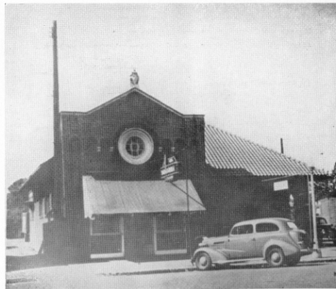
New Station, Chillicothe, built 1912
