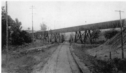
Undercrossing with N & W Railway at Kinnikinik, Scioto Valley
