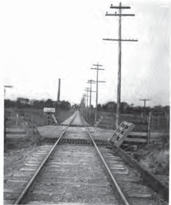
TYPICAL CROSSING, SHOWING CROSSING SIGNS AND GUARDS, SCIOTO VALLEY
