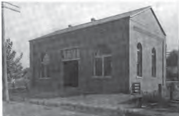
SUB-STATION BUILDING, SCIOTO VALLEY
