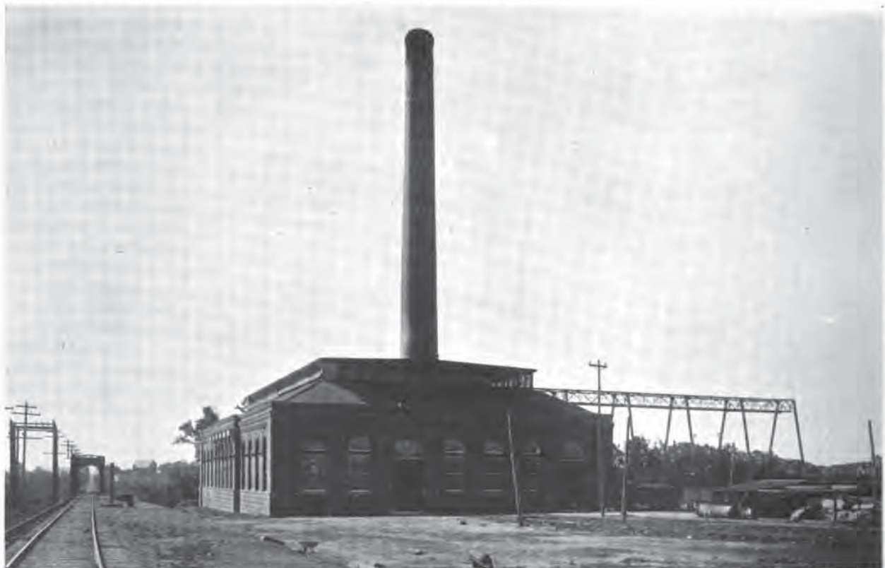
EXTERIOR POWER STATION, SCIOTO VALLEY
