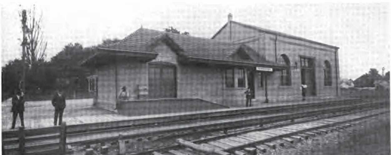
COMBINATION FREIGHT, PASSENGER AND SUB-STATION AT KINGSTON, SCIOTO VALLEY
