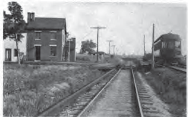
OBETZ JUNCTION, THE JUNCTION POINT OF LANCASTER AND CHILLICOTHE DIVISIONS. THE PASSENGER STA- TION PLATFORM EXTENDS OVER THIRD RAIL— SCIOTO VALLEY
