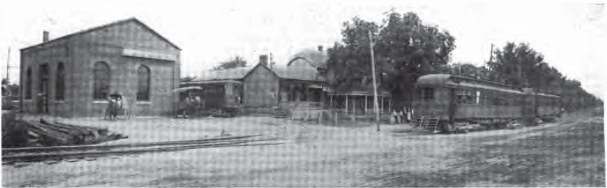
SUB-STATION AND TEMPORARY FREIGHT AND PASSENGER STATION AT CHILLICOTHE, SCIOTO VALLEY
