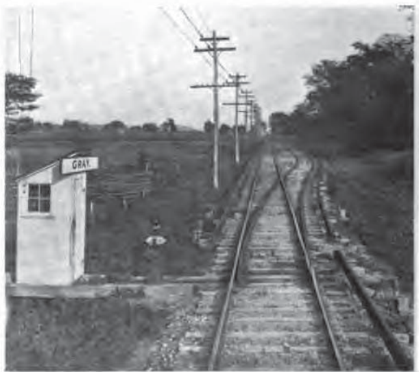
STANDARD TURNOUT, SHOWING SWITCH STAND, TELE- PHONE BOOTH AND THIRD-RAIL CONSTRUCTION AND CONNECTIONS, SCIOTO VALLEY
