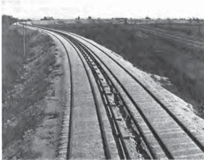
THE "BIG FILL" AT OVERCROSSING WITH H. V. RAILWAY, SCIOTO VALLEY
