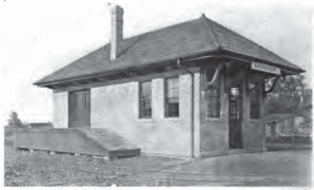
FREIGHT AND PASSENGER STATION AT GROVEPORT, SCIOTO VALLEY
